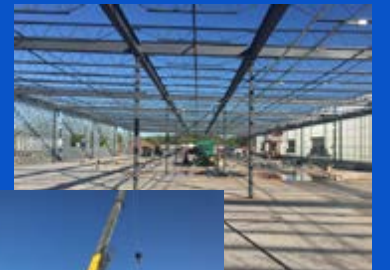
Bonham Elementary Construction
